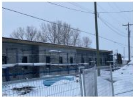
Photo of exterior of new inpatient unit.
